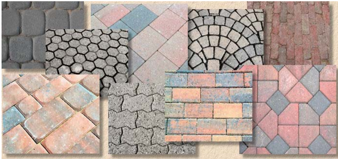
Concrete Paver Blocks Laying patterns
