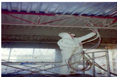
FIGURE 1.5: Spray gypsum based plaster fireproofing being installed.
