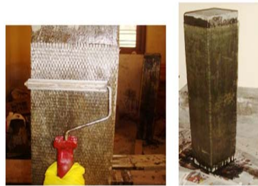
Strengthening by EBR method
