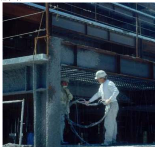
Figure 1.3: Construction worker applying spray resistive material
